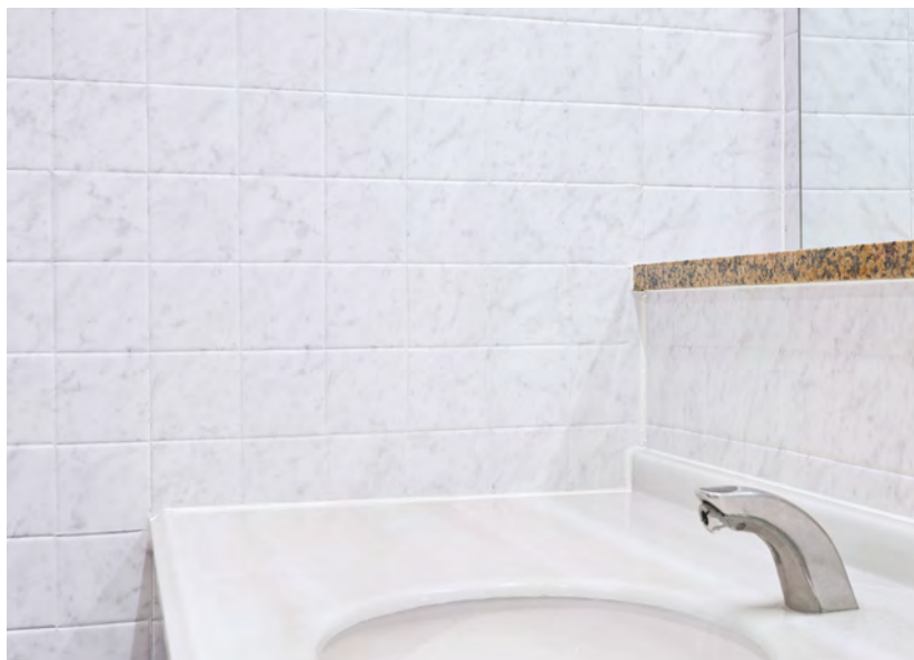
Restroom refurbishment / ST-024TIL
